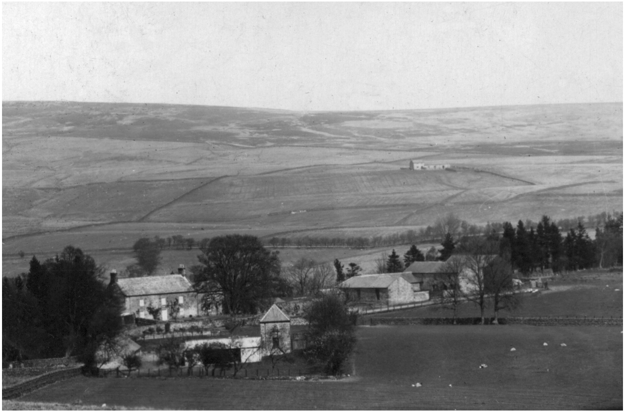
Heathery Hall, far background right, with Redheugh and its dovecote (A0003; A0014) in the foreground.
