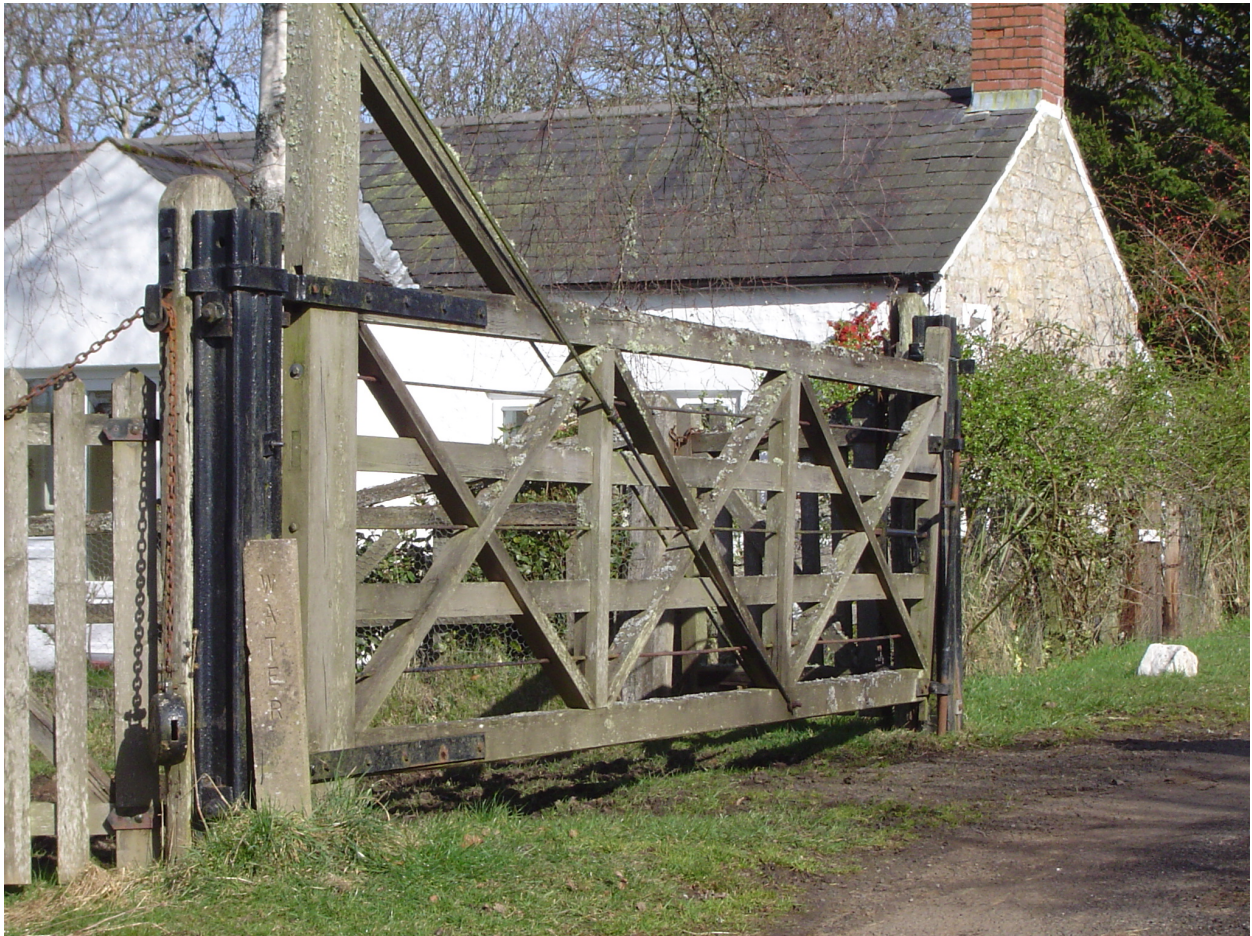
Thorneyburn station gates.
