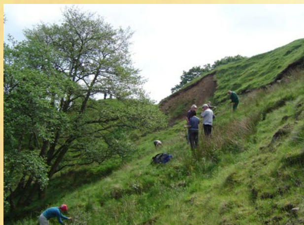
2007 TAG approached English Heritage about deterioration of site; as an interim measure TAG, with help from NNPA volunteer rangers, planted 1200 willow slips in an attempt to improve slope's stability
