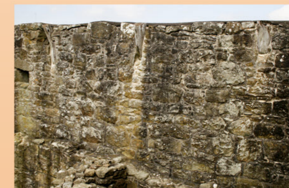
Black Middens remnant roof supports
