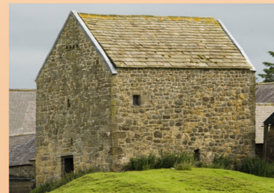
The Hole Bellingham example of a stone-roofed Bastle
