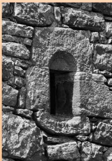
North Gatehouse window possibly re-used from another building
