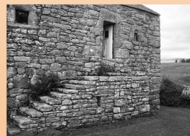
North Gatehouse steps built in two stages; first forming rectangular platform below doorway; lower section added later
