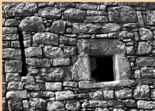
North Gatehouse window and ventilation slit
