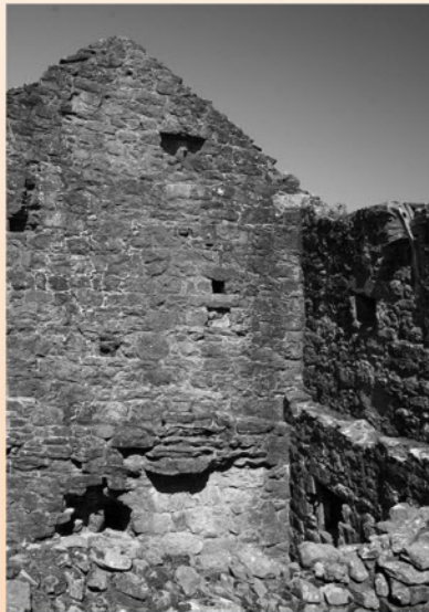
Black Middens 1 interior side walls set back to accommodate floor joists; a surviving roof timber on right; recesses in walls for storage at various levels
