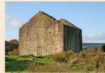
South-east gable wall with original ground floor byre doorway, now blocked
