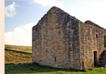
North-west gable wall with small ventilation slit on the ground floor
