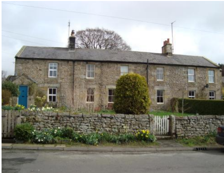
A simple linear terrace at Greenhaugh; stone walls, slate roof, tight verges and eaves, chimneys and rhythmical placement of windows, all tied to the wider landscape with stone boundary wall.
